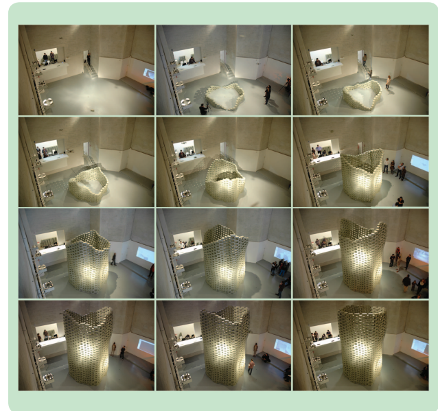
FIGURE 17 Time-lapse photos of the event. The structure was assembled in front of a live audience over four days. From left to right, top to bottom, the height of the structure in layers is 1, 7, 15, 18, 24, 36, 47, 52, 58, 60, 60, and 60.
