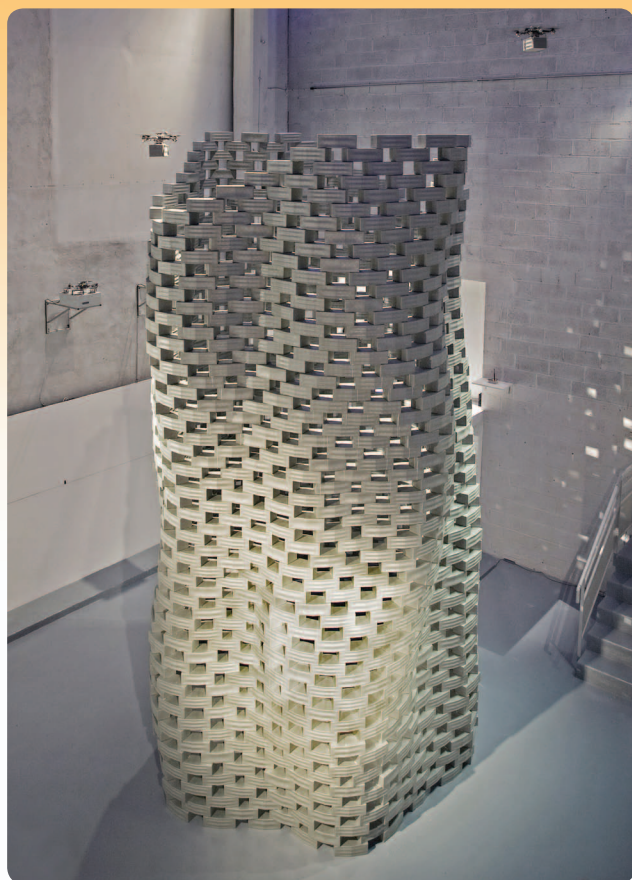
FIGURE 1 The Flight Assembled Architecture installation. The 6-m-tall tower consisting of 1500 foam elements was assembled by four quadcopters in France, 2011. (Photograph by François Lauginie.)
